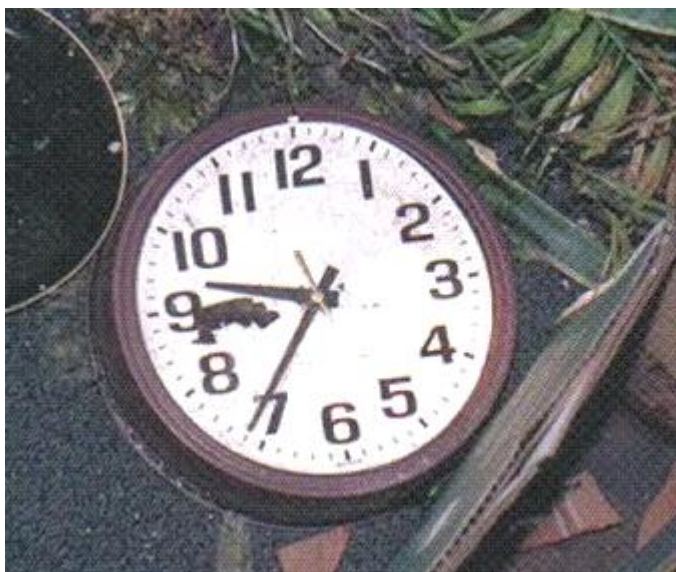
Figure 1: Stopped Clock from Room 3E452 near “Hinge” of Collapsed Floors
